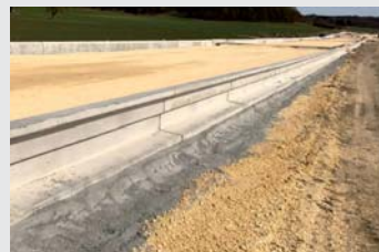
Beton / Concrete Ideal Sondervariante Laubfrosch-/Molchtauglich Special version proof for salamander and tree frog
